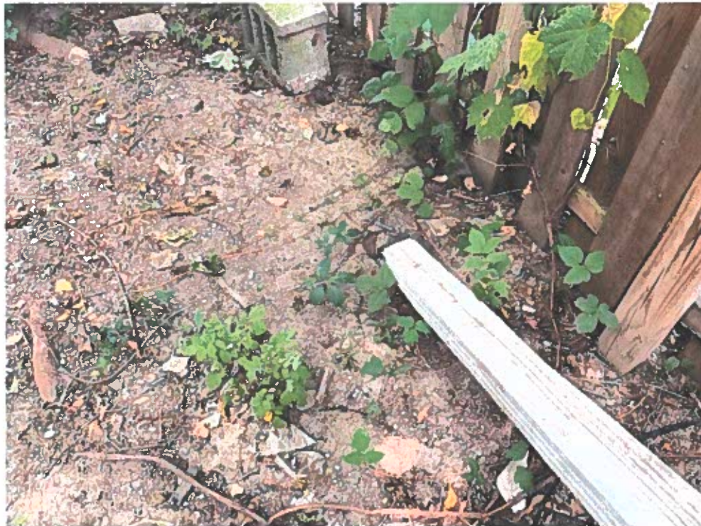
View of roof leader discharge point
