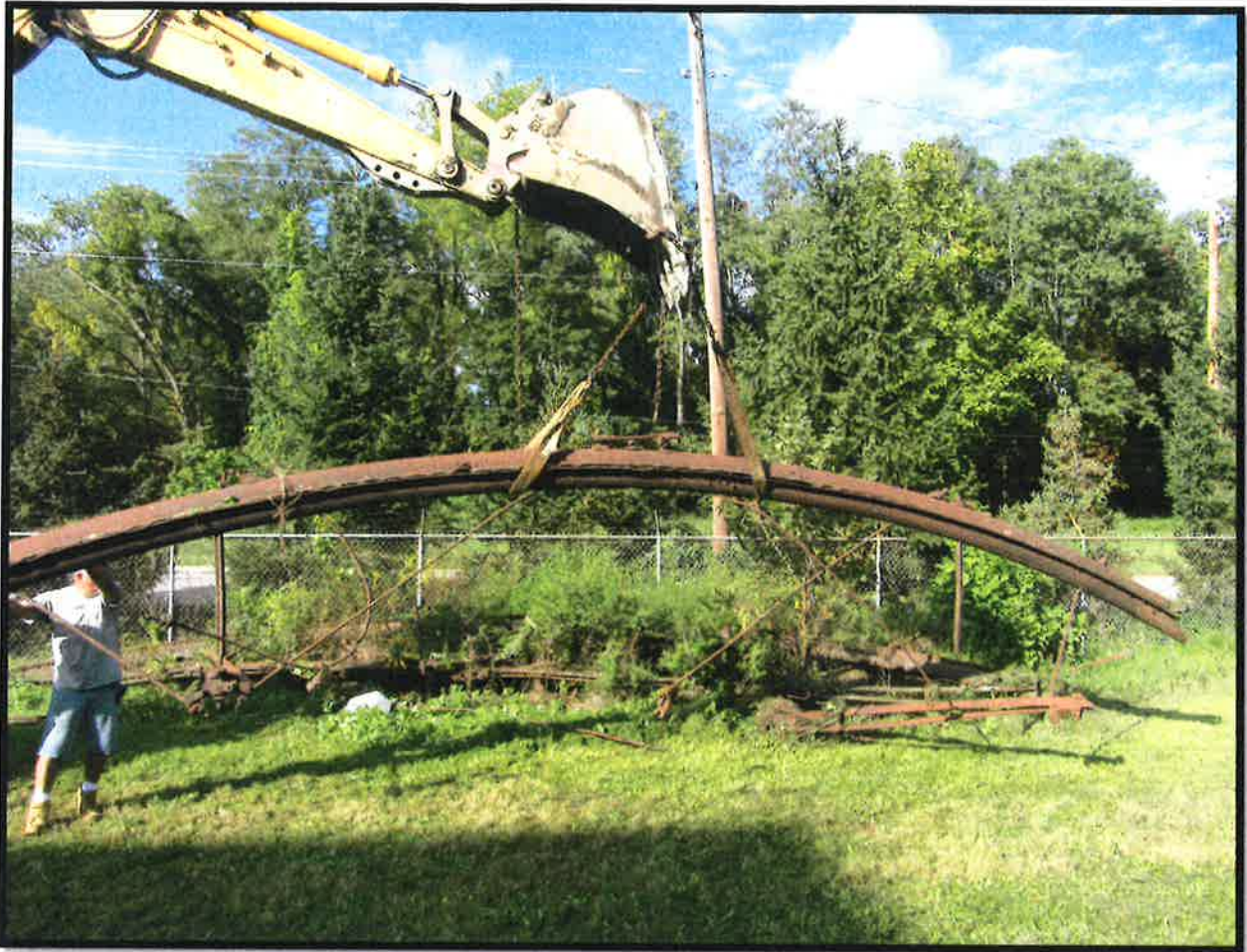
Lifting first arch from pile
