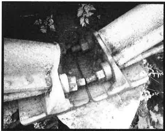
Bridge Seat detail on midstream pier
