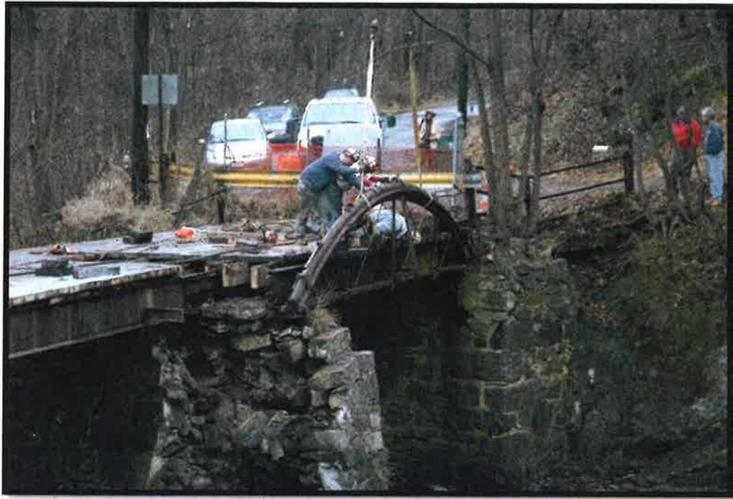
Removing Last Arch
