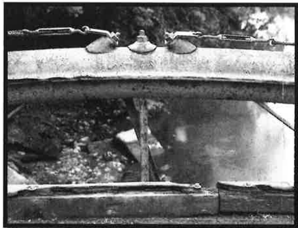
Detail of top chord diagonals & vertical
