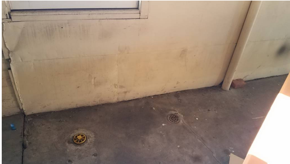
Photo 1: Presumed former bathroom on second floor
