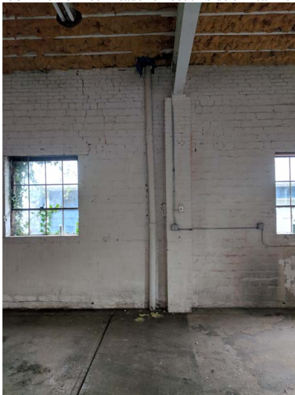
Figure 4 - View of Roof Leader on North Side of Rear Building
