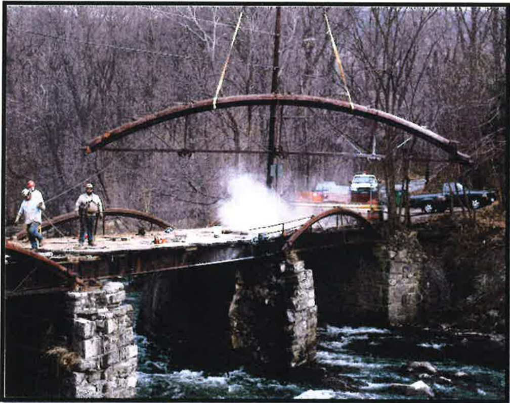
Removing Center Arch
