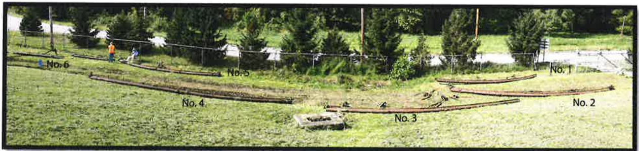
All six arches laid out on the ground
