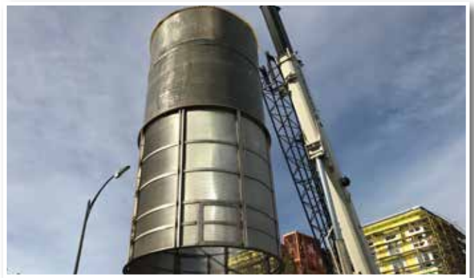
CDS standalone system removes trash and sediment.
