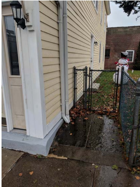
Figure 1 – View of Roof Leader Pipes Located in the Southwest Corner of the Front Building
