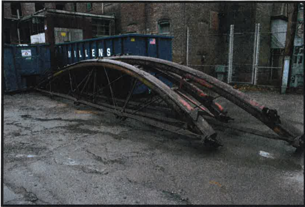
Three arches in temporary storage in seeming good condition.
