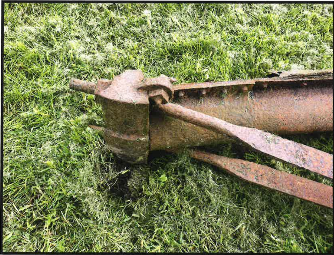
Joint L0 under
