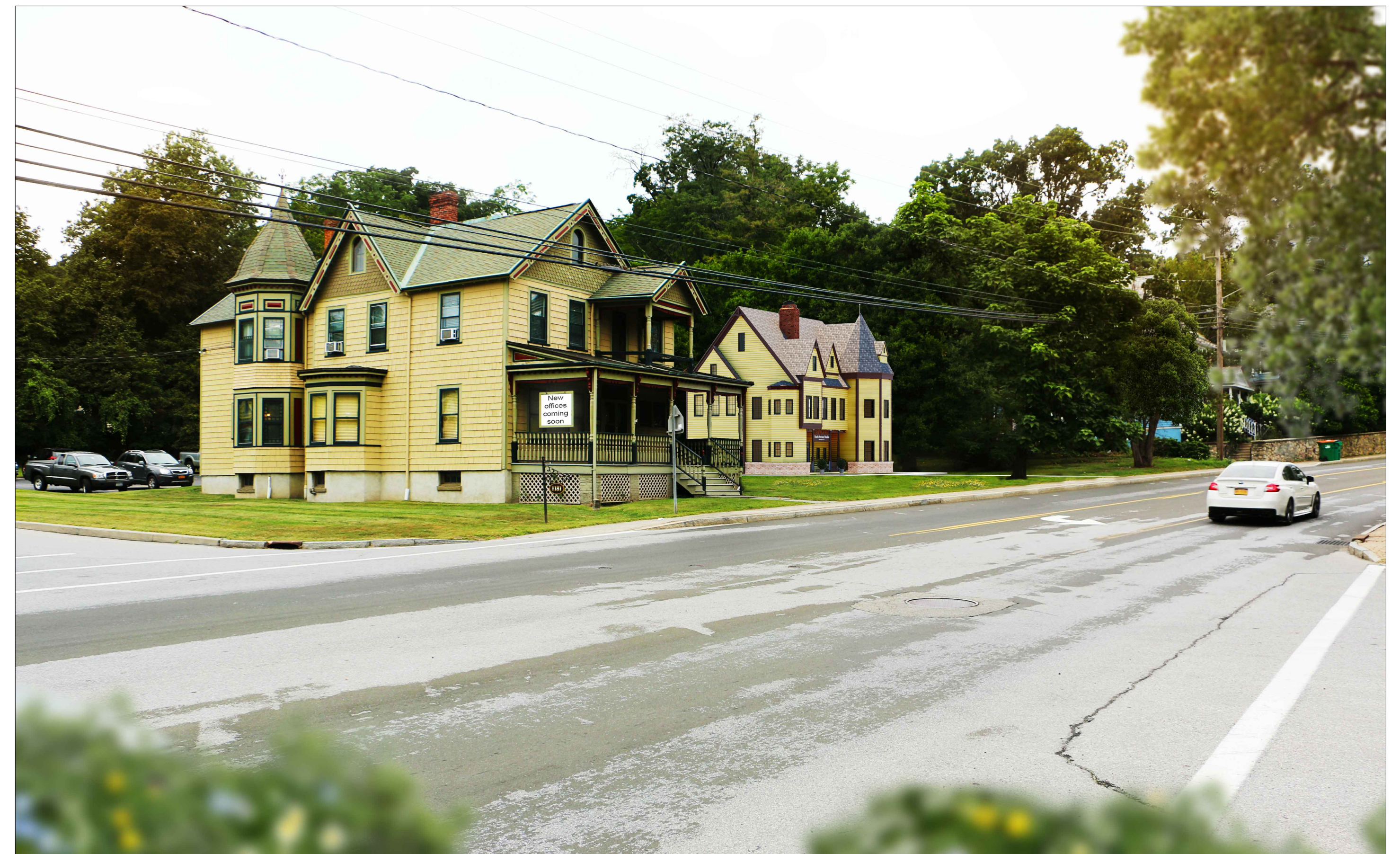
View Looking North
