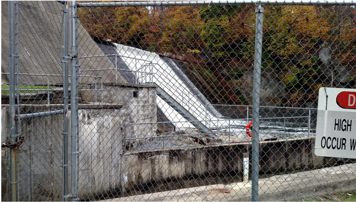
Photo 8: View to the east of the existing dam along Fishkill Creek.
