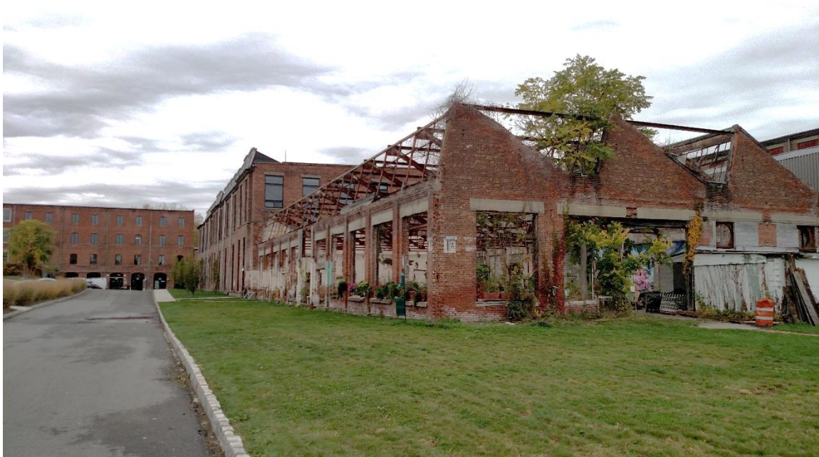
Photo 3: View to the northeast of the Community Garden Building. Building 11 and Building 4 within the Beacon Lofts complex can be seen in the far ground.
