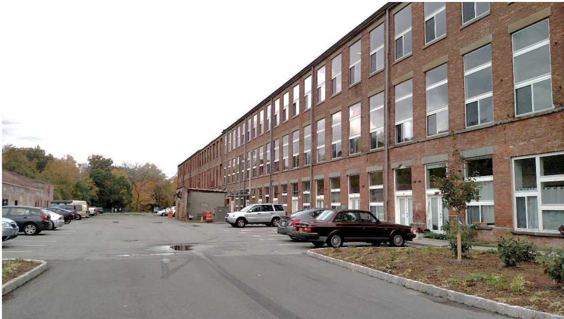
Photo 10: View to the southwest of Buildings 11 (right) and Building 16 (far ground).
