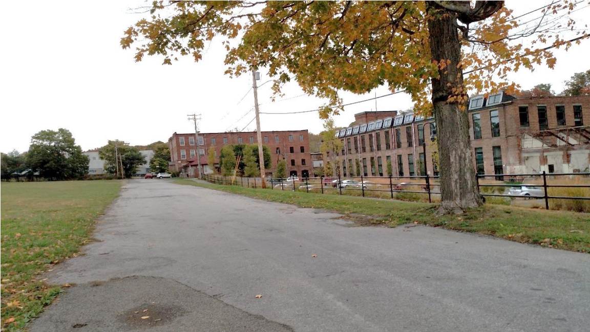
Photo 14: View to the northeast along Front Street. The Beacon Lofts Offices and self-storage building are located at the end of the road.
