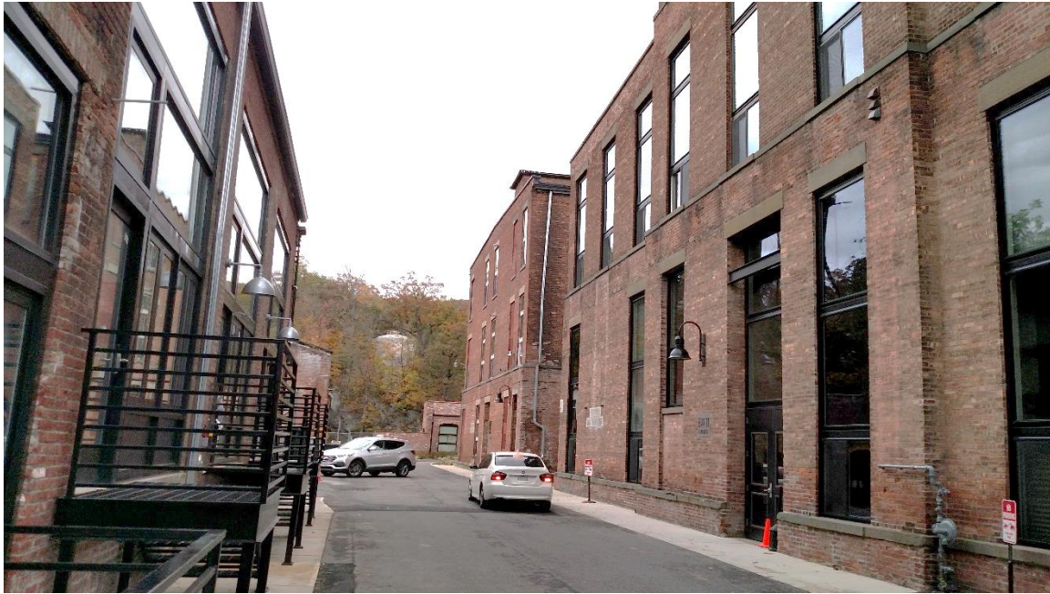
Photo 9: View to the northwest from the hydroelectric facility along Mason Circle between Building 11 (left) and Buildings 1-4 and 19-20 (right).
