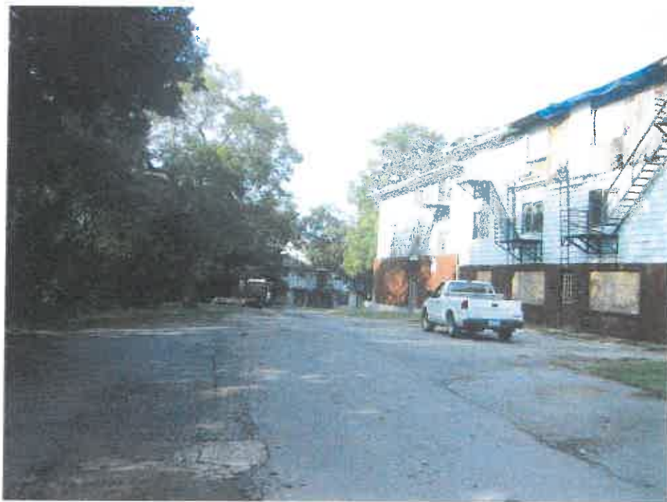
Photograph looking southwest along 2-story frame building
