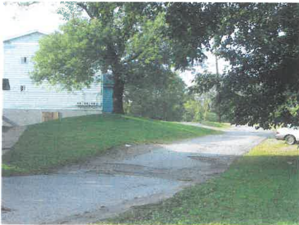
Photograph looking southwest along 2-story frame building
