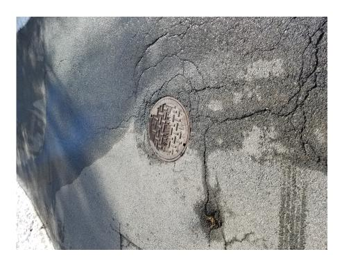
**Manhole Cover @ Davis and North Streets**. Pavement Cracking and settling around the structure and a small sink hole at the bottom center of the photo.
