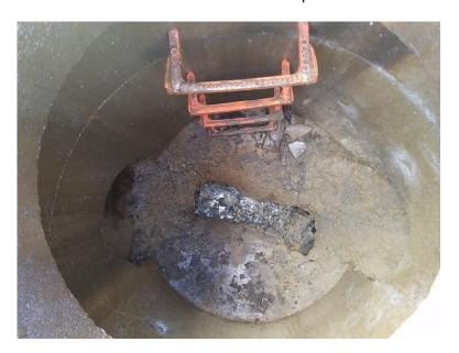
**Manhole with bottom covered in debris.** Manhole that appears it was not completed when installed has mud and debris covering the bottom and partially blocking the troughs. Sewer mapping shows 3 pipes at this location.
